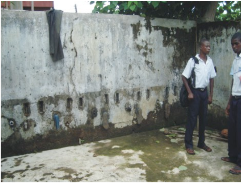
wall showing where the wash-hand basins used to be
