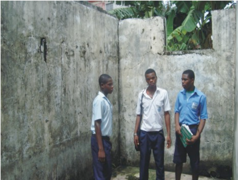
wall showing where the showers used to be
