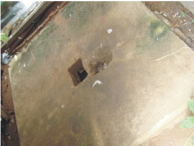
inside the pit toilet
