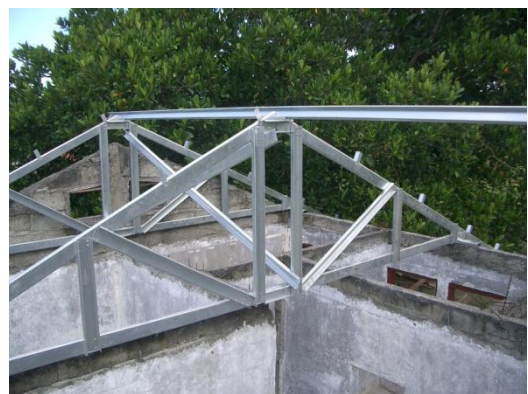
Roof trusses on houses
