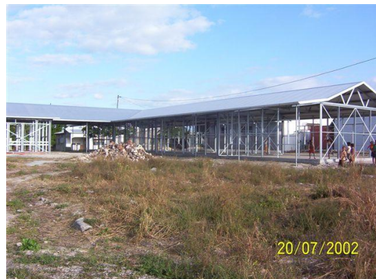
The training centre under construction
