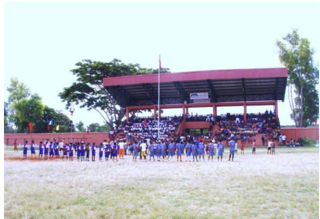
Baucau grandstand, re-roofed and refurbished by ETRP, on Independence Day celebrations.
